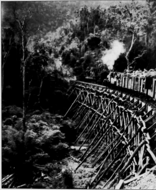
The trestle bridge near Kensoyak.
